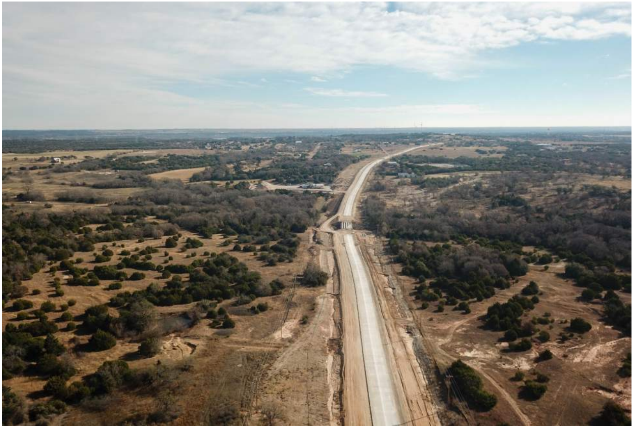
Eastloop Phase III Construction Activity (Looking East from Upper Denton Rd.)
