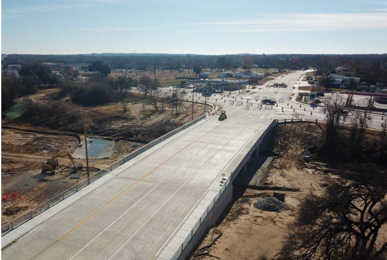
FM 51 Construction Progress (Looking South at SH 199 Intersection)
