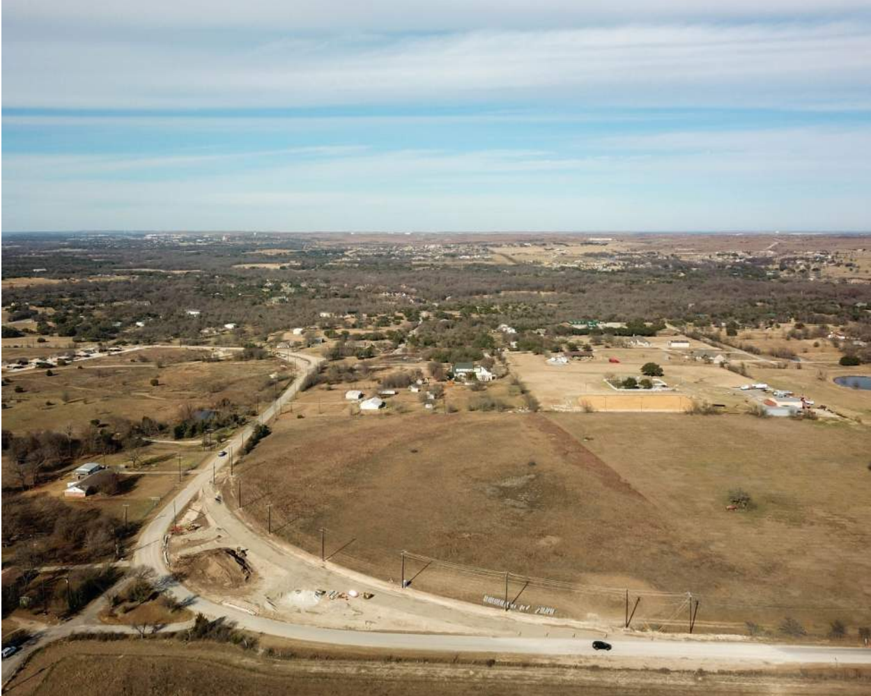
Kelly Road Improvements
