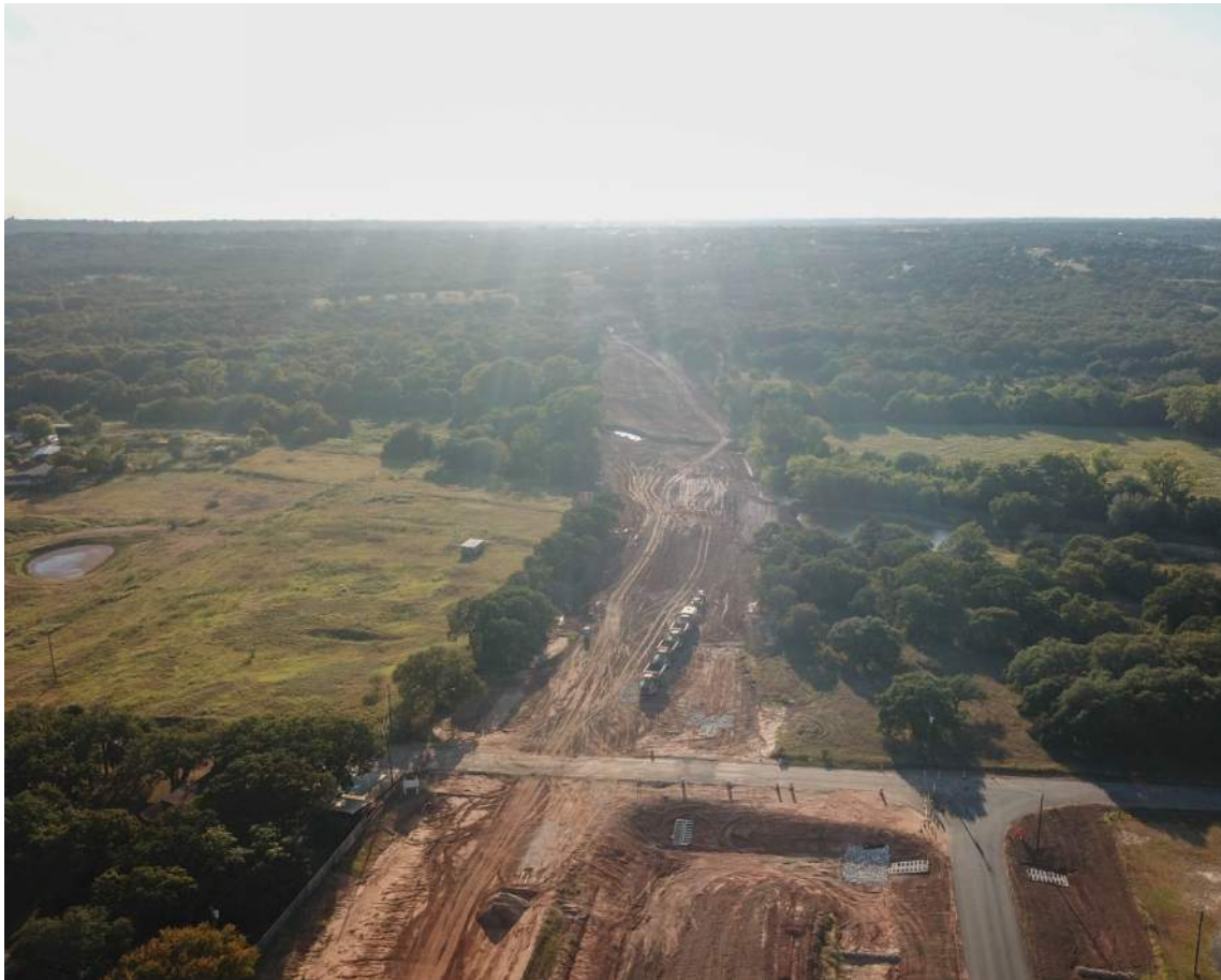
Eastloop Phase III Construction Activity (Looking West from FM 730)
