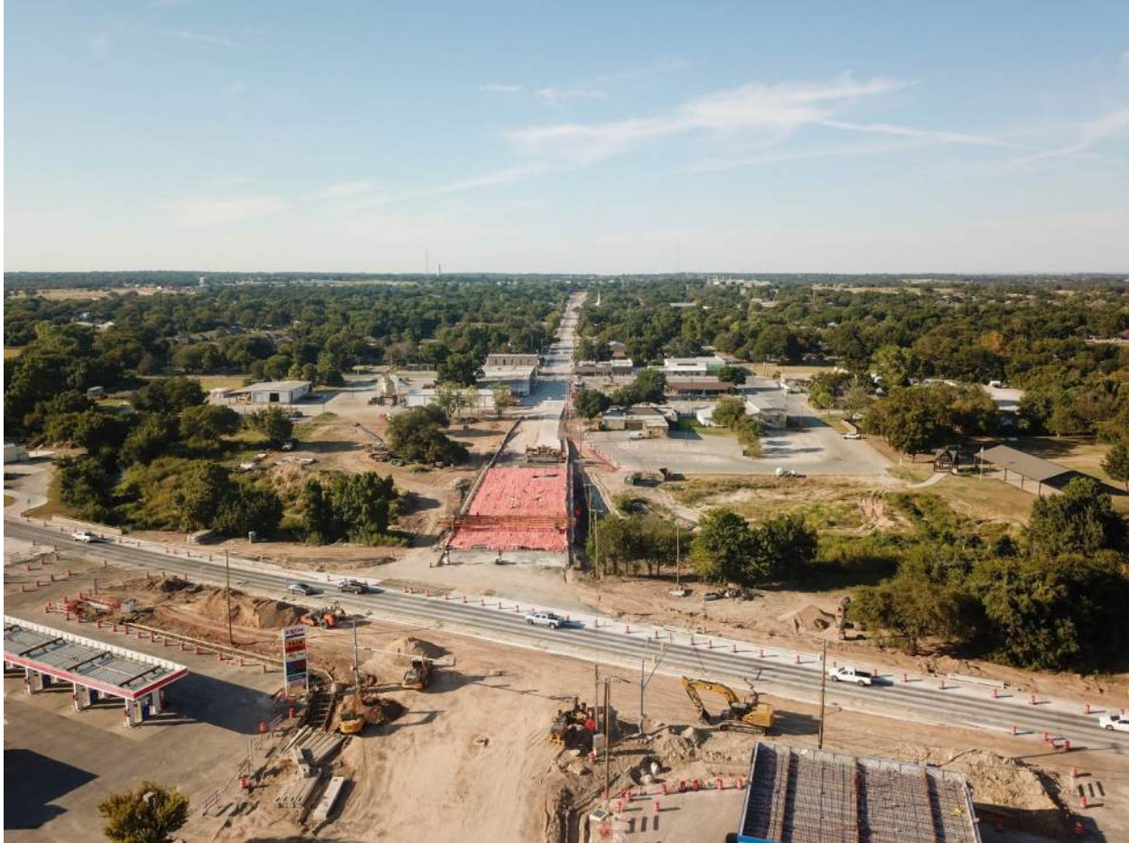
FM 51 Construction Progress (Looking North from SH 199)
